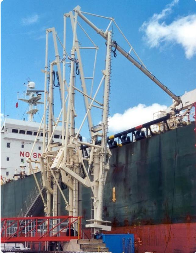
The B0030 marine loading arm is preferred when loading/unloading sea-going tanker ships and its capability has been proven .has been proven with many years of trouble free operation world-wide.
